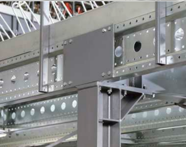
Detailed views of the platform support construction
